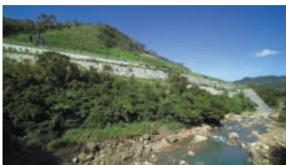
>石碇-加勁擋土牆
