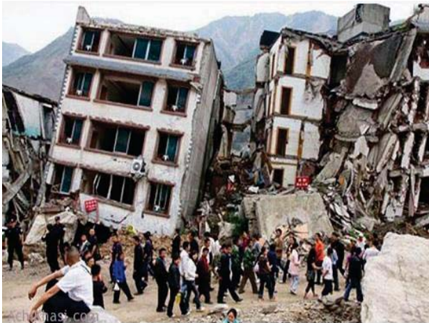
Building collapse in Nepal
